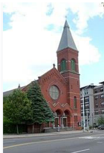
Brick Presbyterian Church in suburban East Orange, New Jersey
