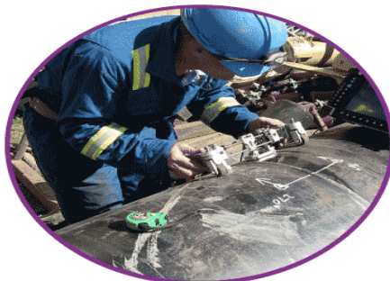
Detection of cracks
